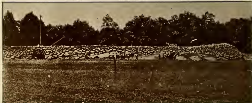
Playstead Overlook under construction, circa 1886.
